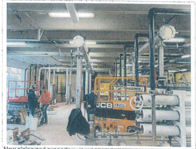
New piping and supports
