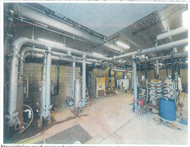
New piping and supports
