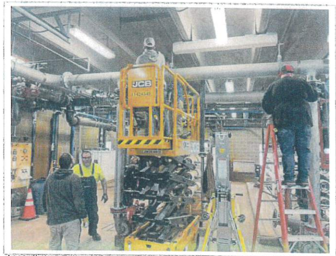
Installation of new piping
