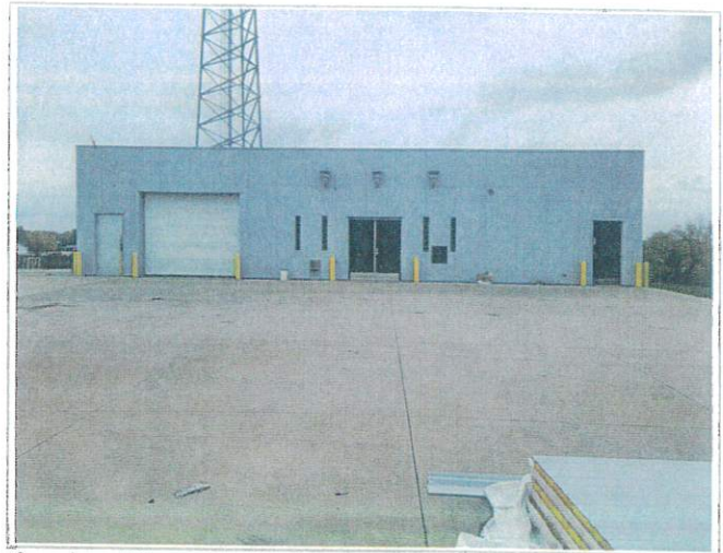
Overview of the south side of the building
