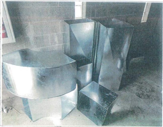
New MUA ductwork has been fabricated and prepped to be installed
