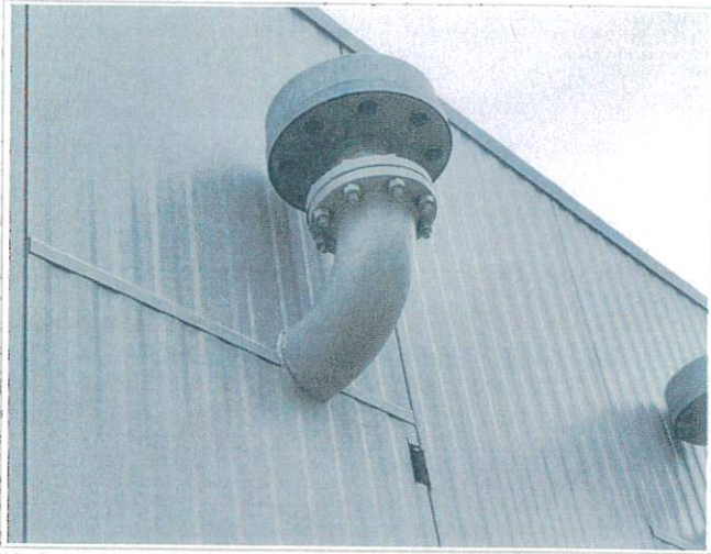
Horizontal seals have been caulked and all penetrations
