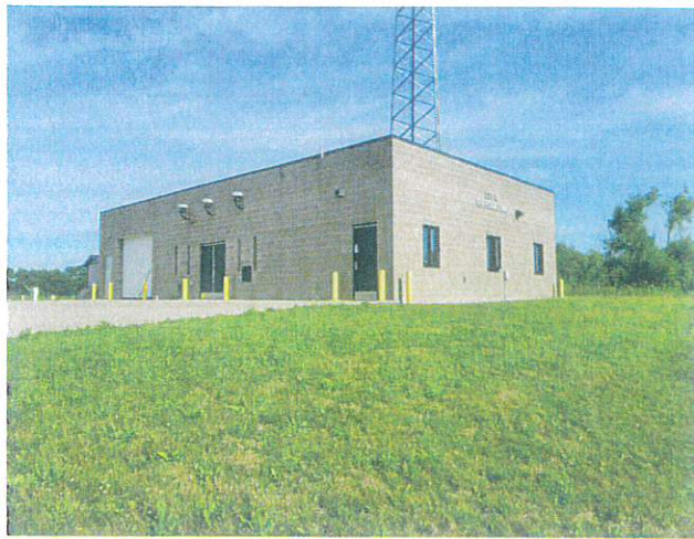
Overview of the building from the SE corner of the property. Building signage and other exterior items have not been removed and it appears the roof is untouched.
