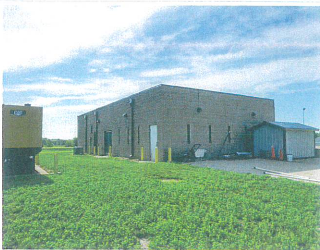
Overall view of the building from the NW corner of the property.
