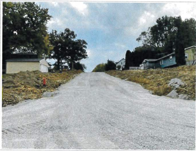
PCI has cored out and graded with road stone - looking east up Third Street from Washington intersection
