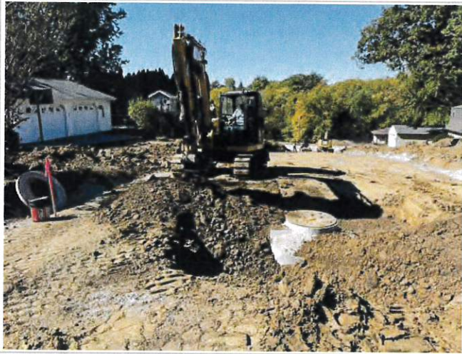
Carter & Associates backfilling new sanitary manhole 30 located just west of Glasgow and Third Street
