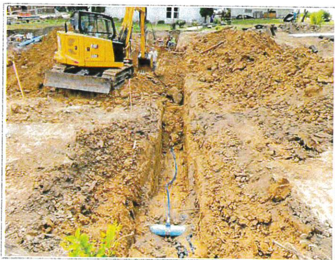
Water services being worked just west of Washburn
