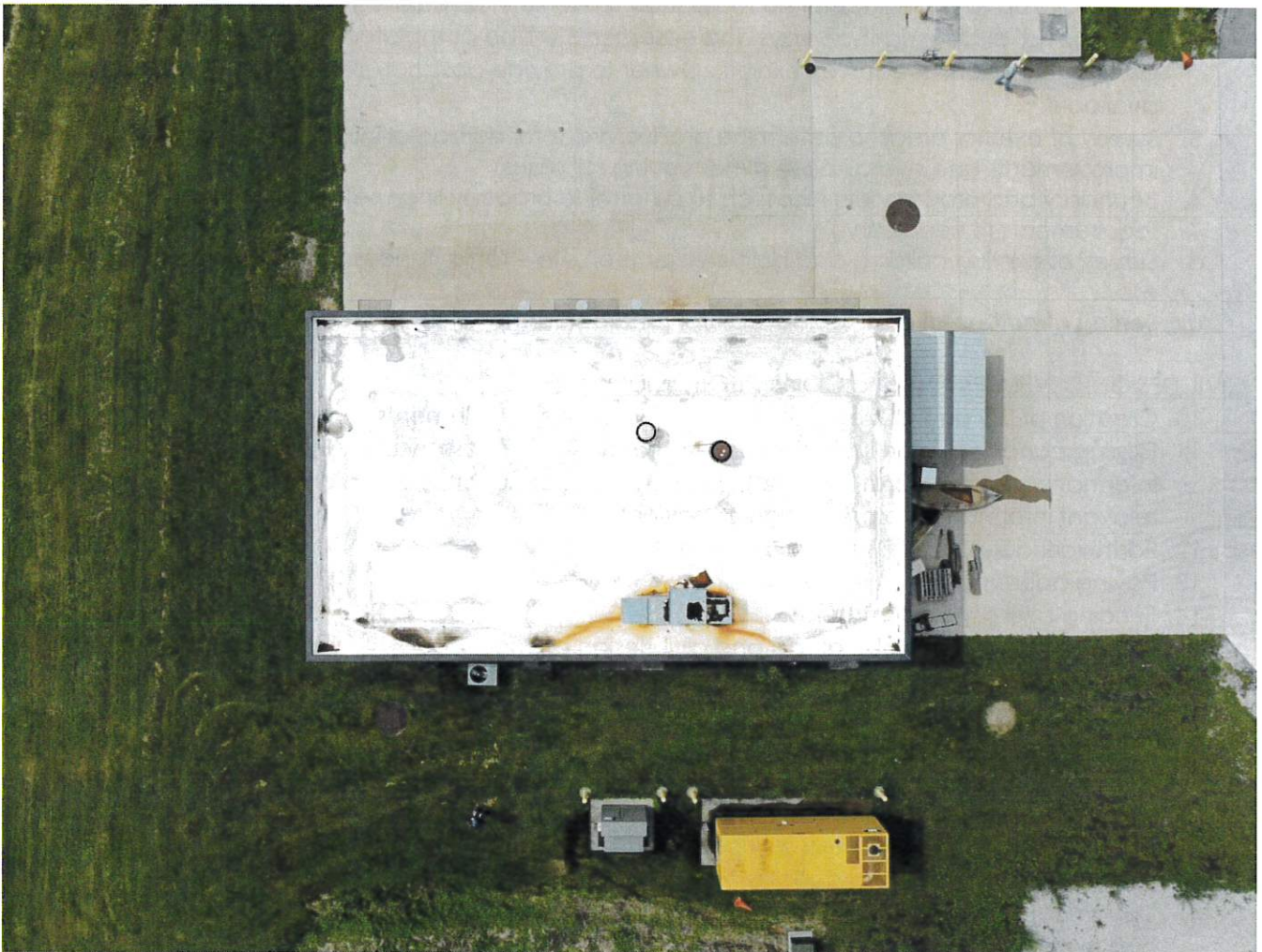
image of WWTP during PCA investigation
