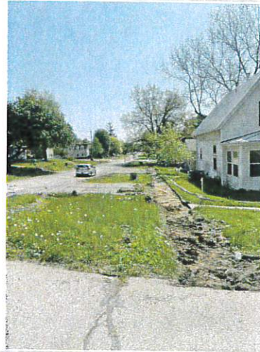
3rd & Greene, looking east down south sidewalk removals along 3rd
