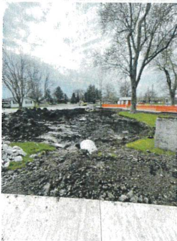
NE corner of site looking south, overview of the rain garden being backfilled and prepped for final F.E.S. and plantings
