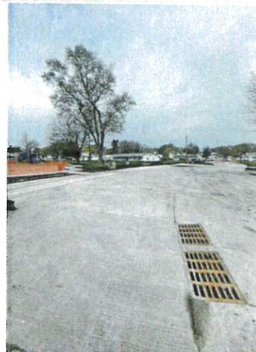
Overview of the west side of S Hickory along the park - shows parking and sidewalk has been poured and finished along the east side of the park since last reporting
