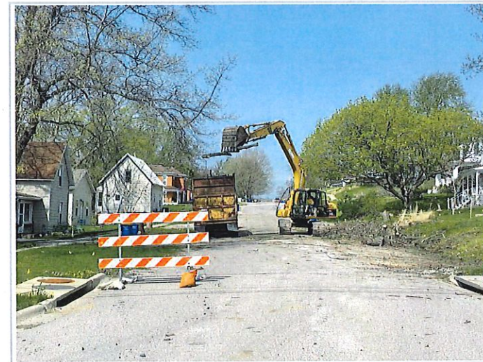
Tree debris being removed throughout the project
