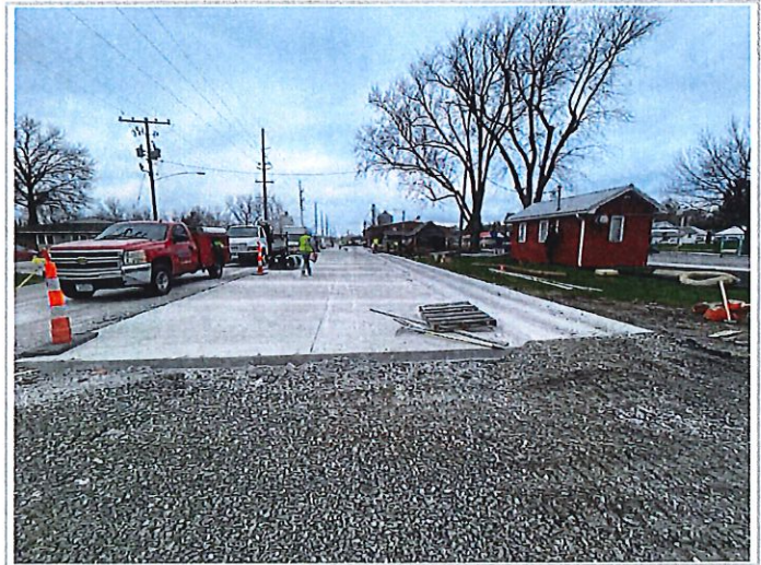
SE corner of site looking West over River Street parking and sidewalk.
