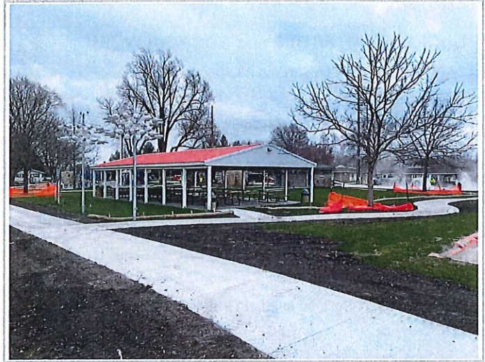
NW corner of site looking over completed sidewalk along 1st Street and West side of project.
