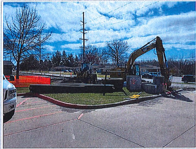
Maxwell materials being stored and staged onsite
