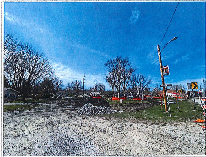
NE Corner of site
