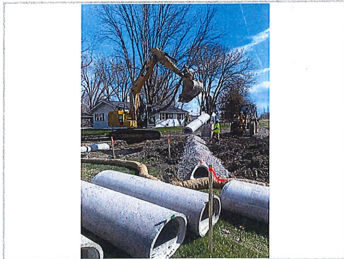
Maxwell installing storm line PR-103.
