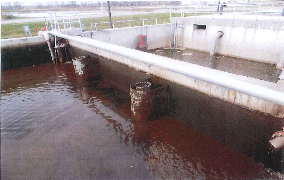
SBR 1 During Fill
